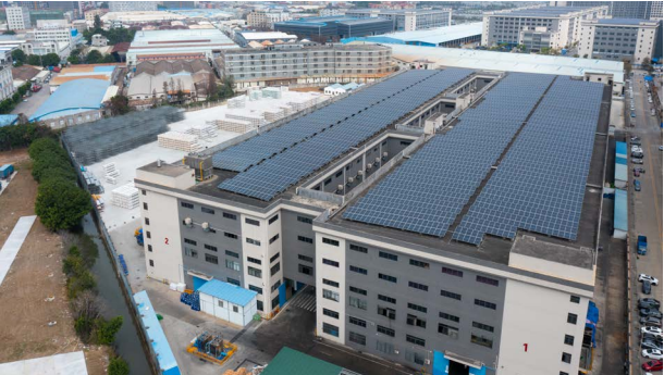
Chongkou Factory Foshan, China
