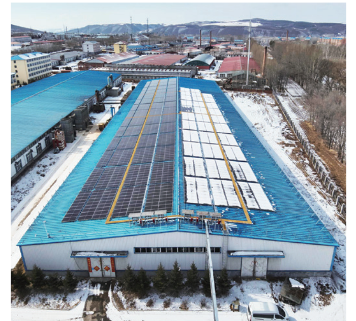
Mulingke Kemian Factory Roof Solar Power Station
