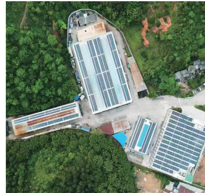
Ducheng Roof Solar Power Station
