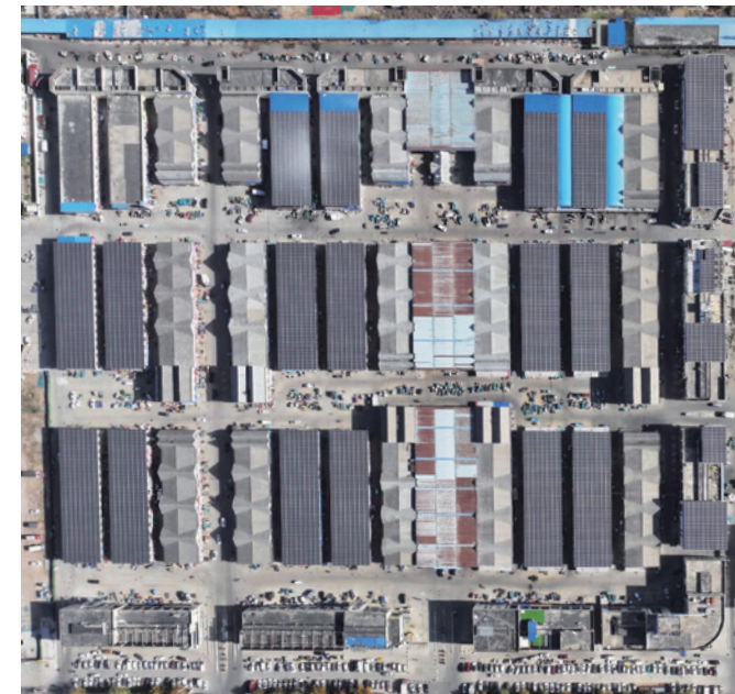
Huanghuai market Roof Solar Power Station
