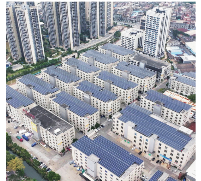
Hongyu Logistics Park Roof Solar Power Station
