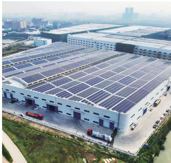
Haitian Roof Solar Power Station
