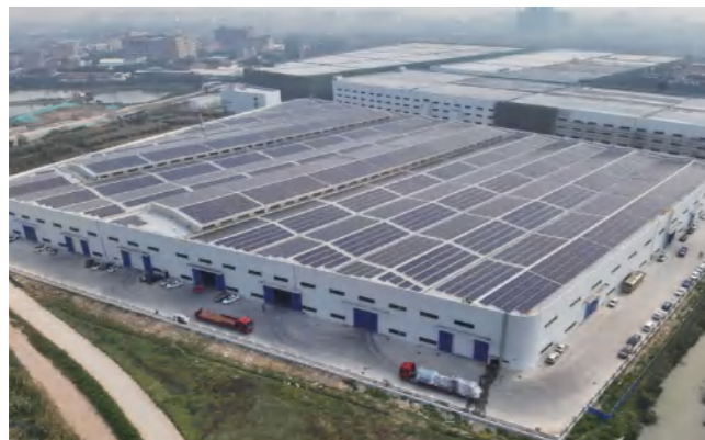
Foshan Haitian Roof Solar Power Station
