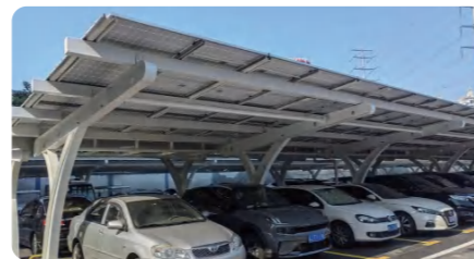
Waterproof PV carport
