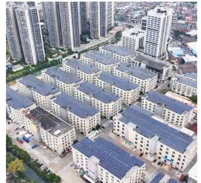
Hongyu Logistics Park Roof Solar Power Station
