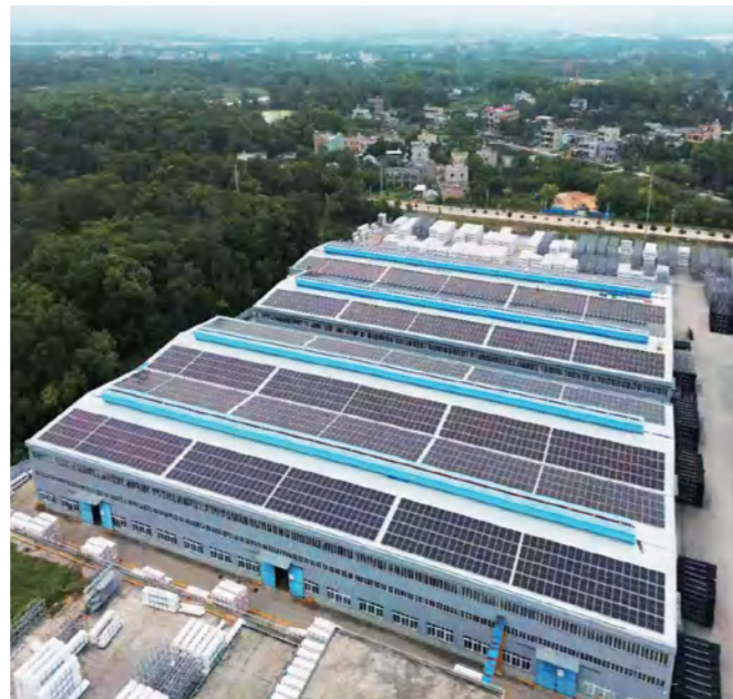
Dingan Roof Solar Power Station
