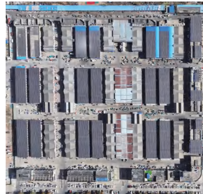
Huanghuai market Roof Solar Power Station
