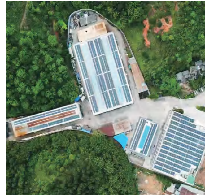
Ducheng Roof Solar Power Station
