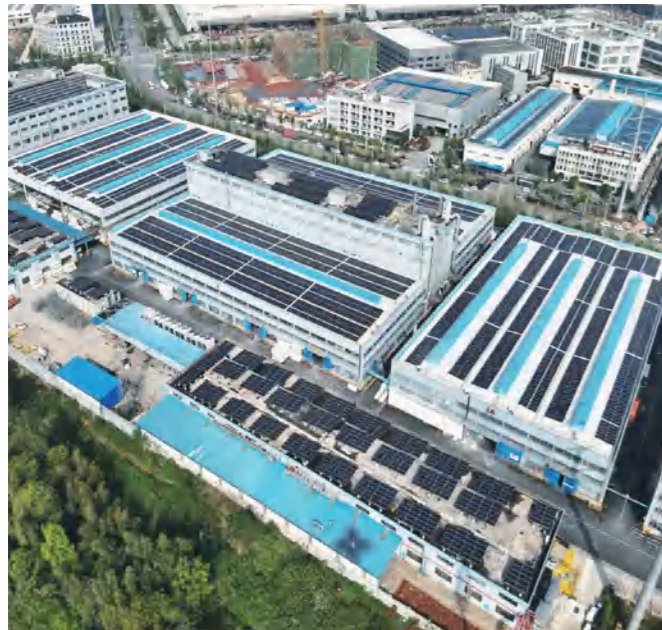
Changsha Roof Solar Power Station
