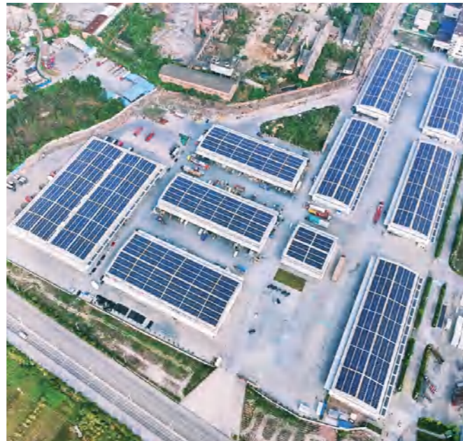
Maoming Logistics Roof Solar Power Station
