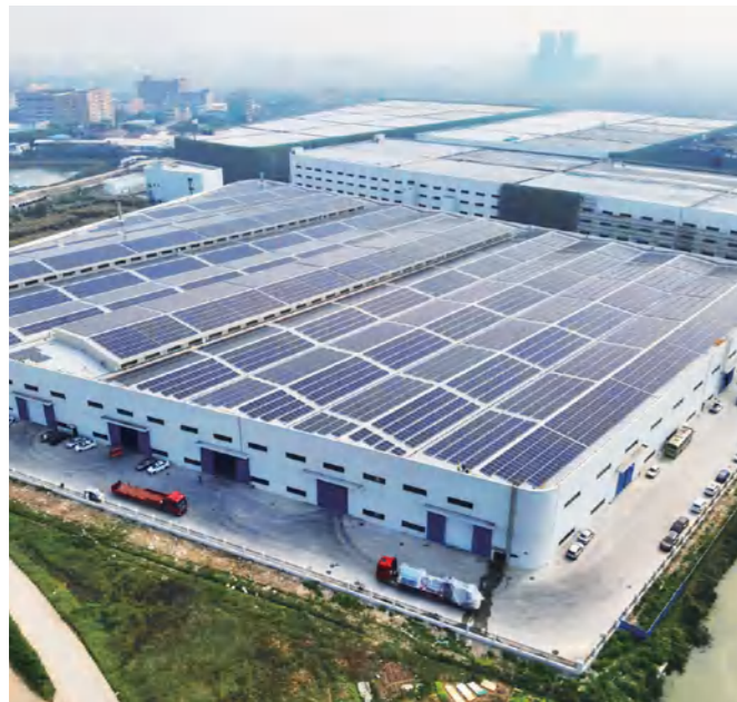
Haitian Roof Solar Power Station
