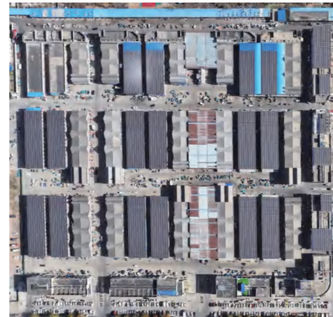
Huanghuai market Roof Solar Power Station
