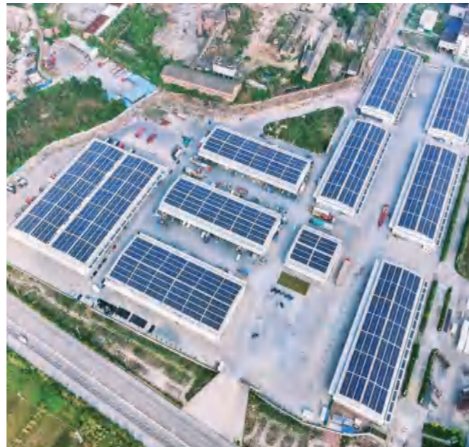
Maoming Logistics Roof Solar Power Station
