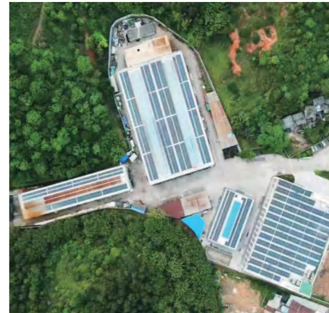
Ducheng Roof Solar Power Station
