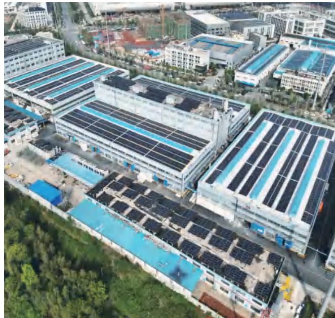
Changsha Roof Solar Power Station
